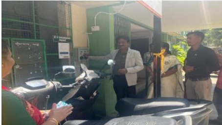
Installation of EV charging unit
