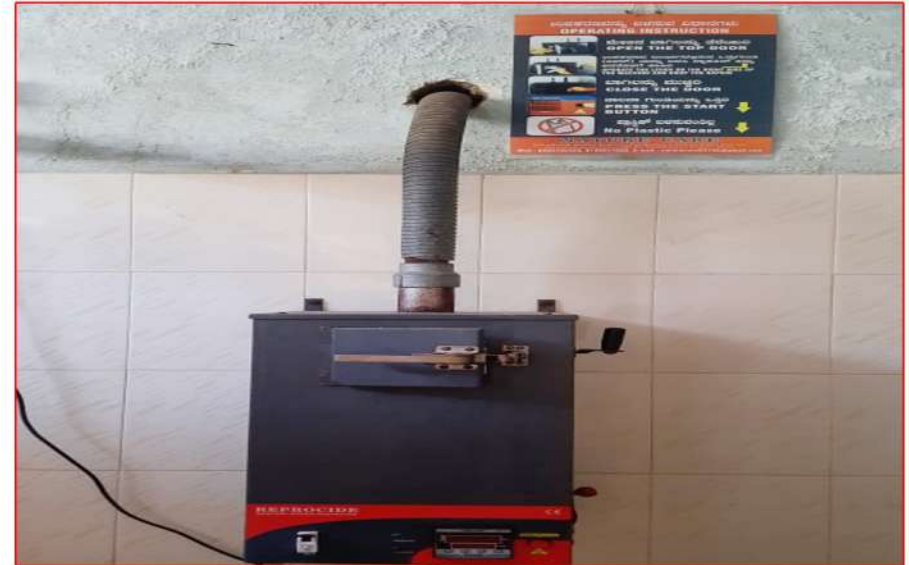
Electrical Sanitary Pad Incinerator
